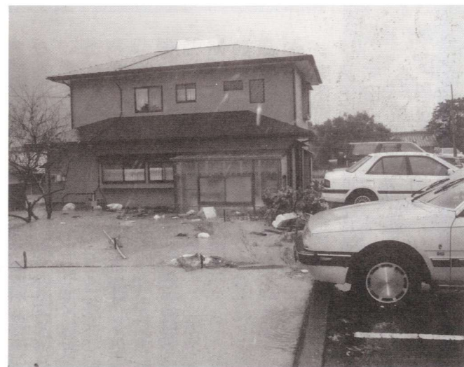
▲役場下職員駐車場も冠水間近
